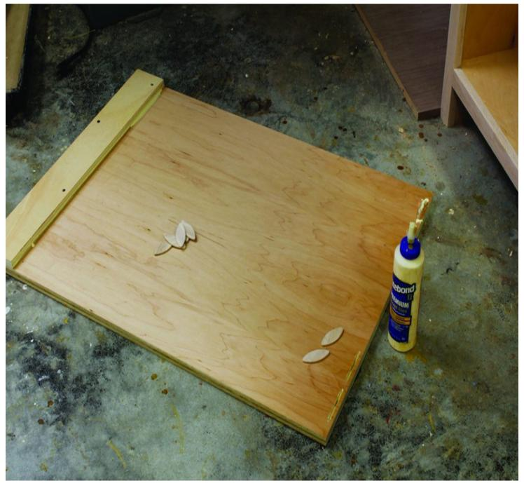
Glue guide. Apply a bead of glue to the top edge of the spacer and where the biscuits will go. Don't waste your time or glue on the pre-finished surfaces; it won't bond to them.
