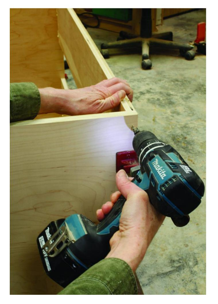
Drill, then screw. Predrill for the screws using a bit just smaller than the shank of your screws. Countersink to prevent breakout. Insert screws with a driver.
