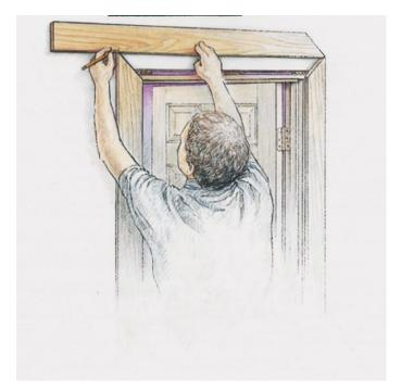
Don't measure: It is more accurate to mark trim in place than to measure and then transfer numbers. It's easy to misread a ruler or to confuse numbers while walking to the saw.
