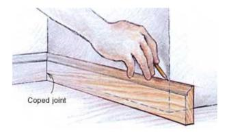
Fit the more difficult end before cutting to length. In this case, the left side is coped and the fit is checked before the miter is marked.
