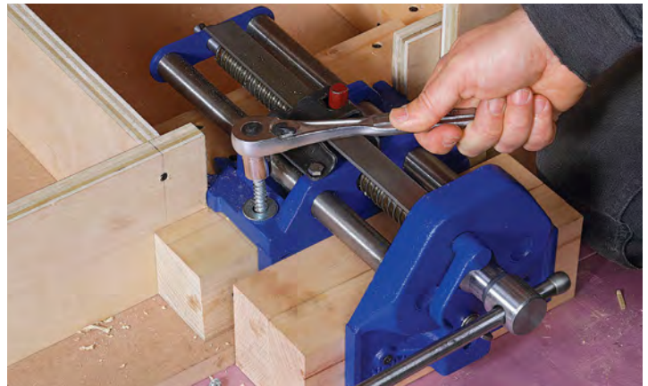
Lag bolts and washers secure vise to bench. These need to be thick, coarse bolts to hold the heavy vise in place. Pre-drill large enough holes for them to avoid splitting the blocking.
