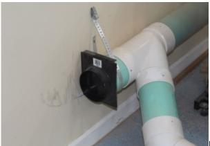
**Extra ports**. When you set up your ductwork consider installing additional ports at logical locations for possible future expansion. It is easier to do it now rather than pulling your ducts apart later. You can add a blast gate so you are ready to go, or simply place a cap on the pipe which is a bit cheaper. This can also provide a nice cleanout in a convenient location should something ever get lodged in your ductwork.
